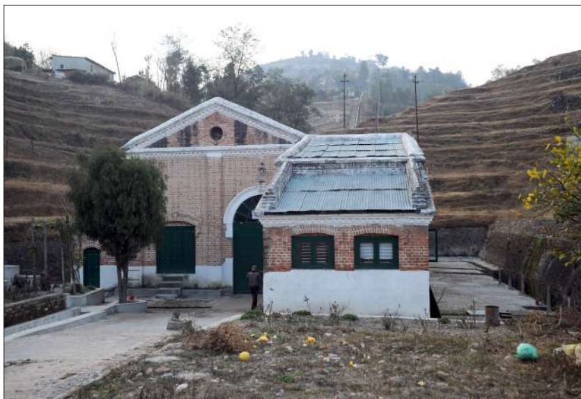
First Hydropower Plant of Nepal, Pharping, Kathmandu
