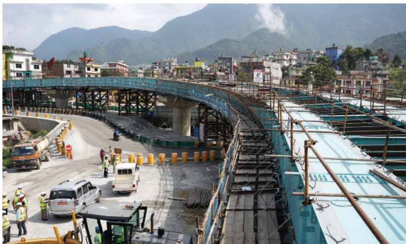
Flyover Towards Nagdhunga Tunnel, Kathmandu
