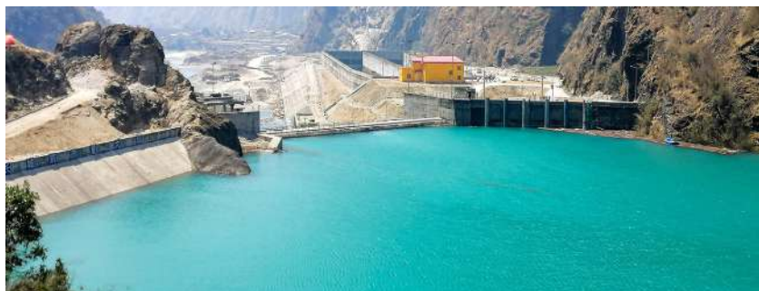
Upper Tamakoshi Hydropower, Dolakha
