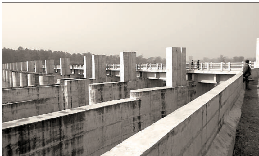
Sikta Irrigation Project
